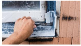
7. Install the AEROSANA FLEECE sub-sill flashing
