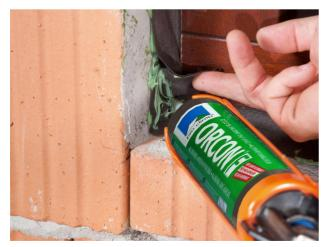
**6. Stick the corners** Stick the folded corners together using ORCON F. The tape can then be plastered over more easily later on.
