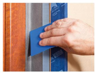
**5. Rub the tape firmly to secure the adhesive bond** Rub firmly using the pro clima PRESSFIX application tool to secure the adhesive bond.
