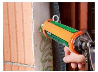
**4. Apply adhesive to surface** Apply a line of ORCON F joint adhesive to the reveal in a compact zig-zag pattern.
