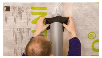
**1. Pull the grommet over the pipe and align it** Select a grommet to suit the diameter of the pipe, pull it over the pipe, guide it as far as the subsurface and align it as desired.
