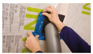
2. Stick the grommet and rub it firmly to secure the adhesive bond
