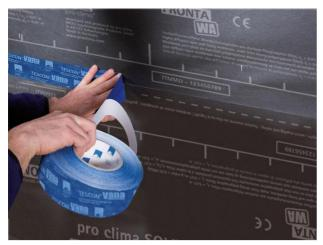
5a. Alternatively: Taping over the overlaps with TESCON VANA
